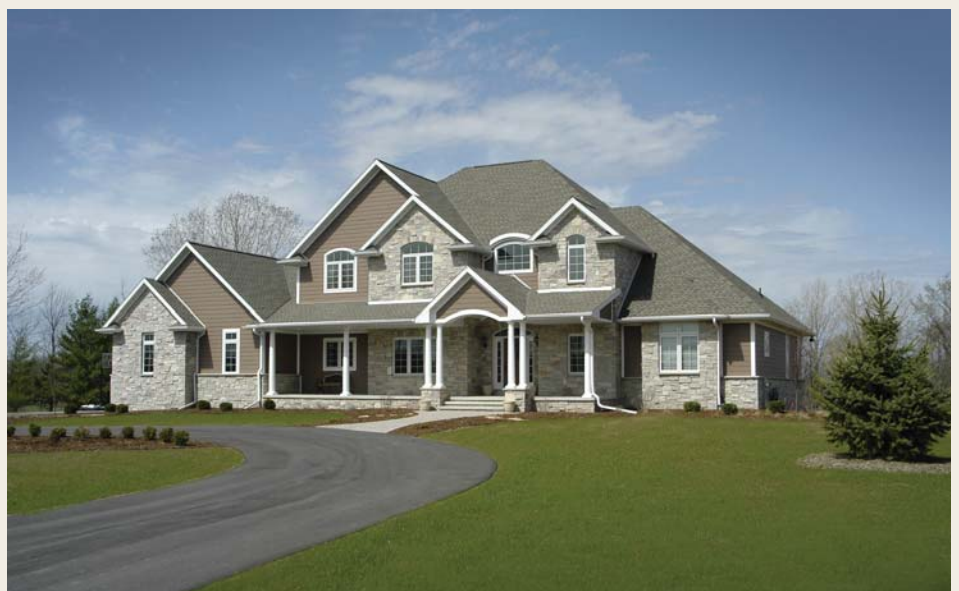
With this two-story home Scott wanted to create a little west coast style while maintaining the Midwest warmth. © Sanderson Photography, Inc.
